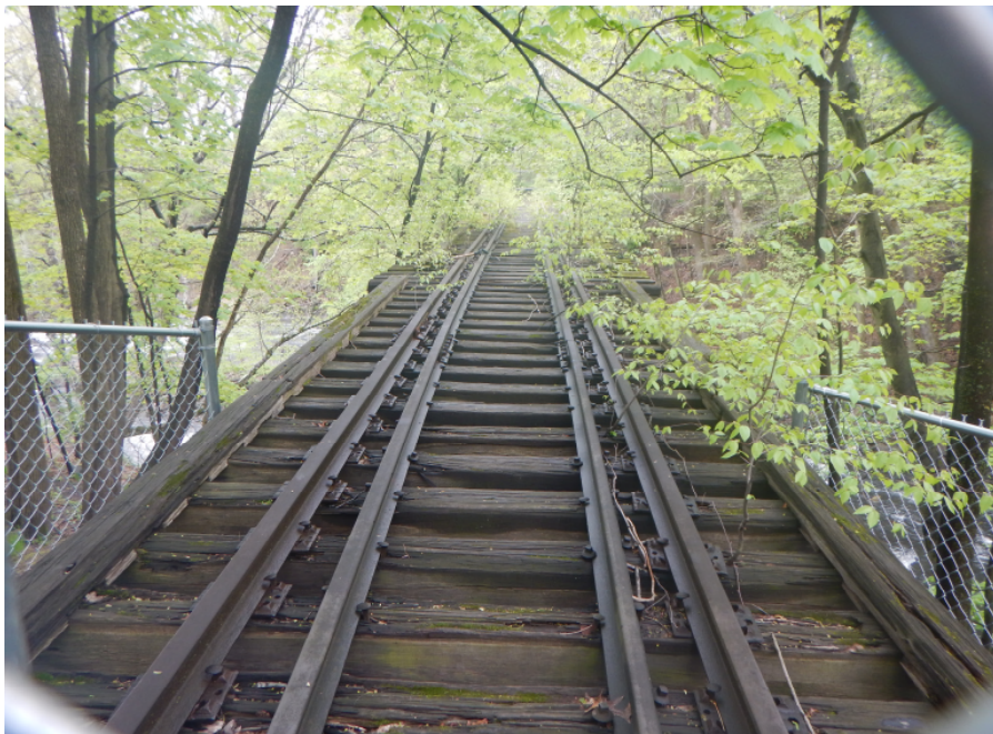
Photo 4: Track, from North Approach to bridge, Looking south.
