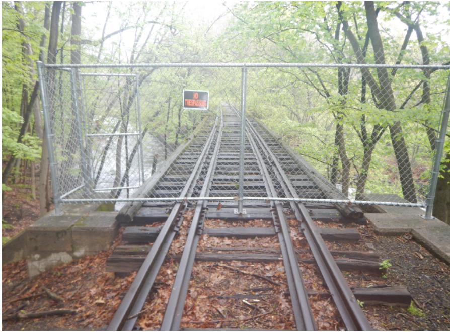
Photo 3: Track, from South Approach to bridge, looking north.
