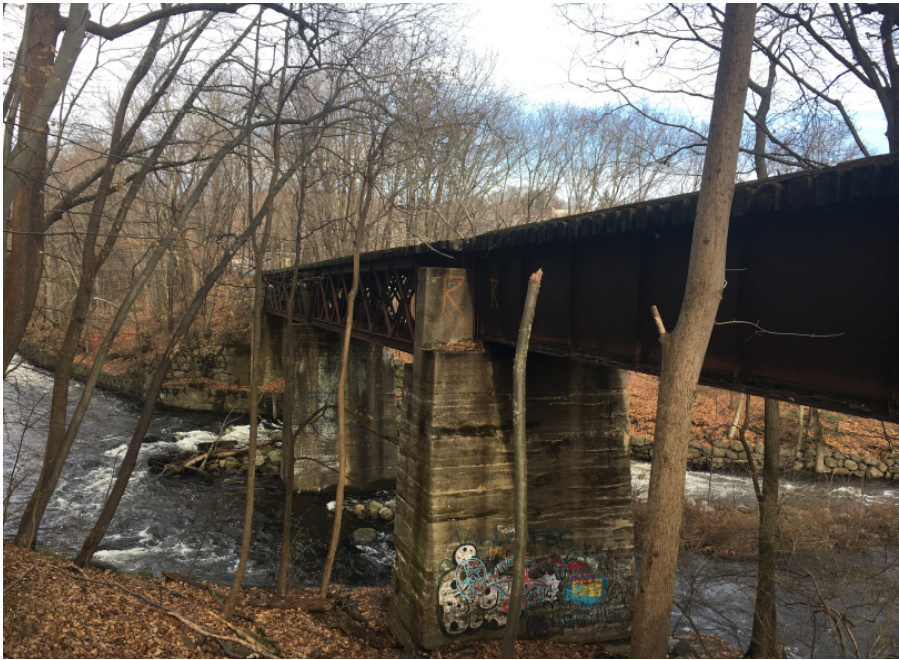
Photo 2: West Elevation, looking northeast.
