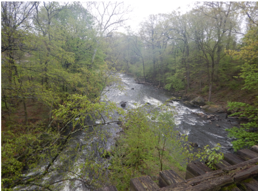
Photo 6: Downstream Channel, looking east.
