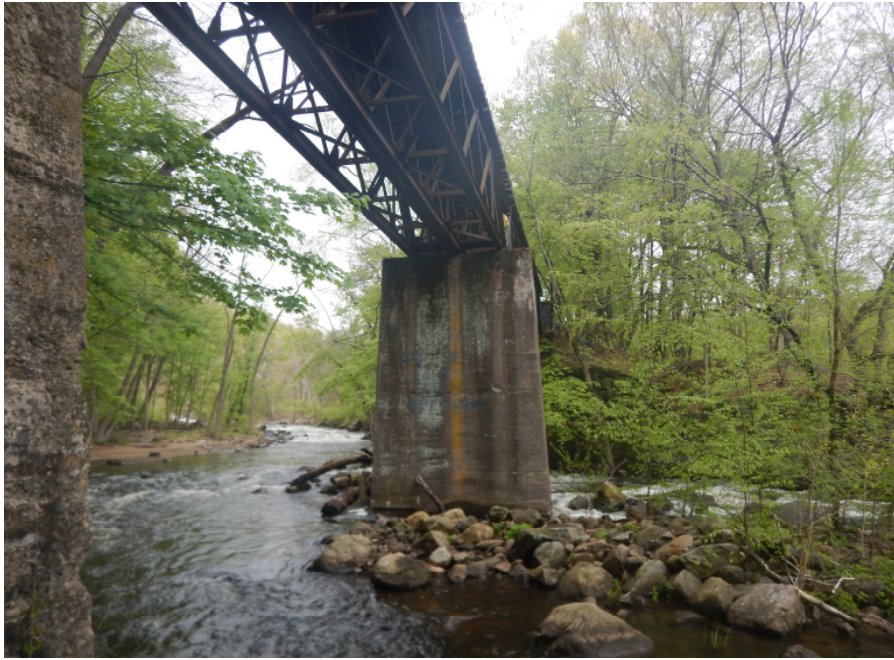
Photo 5: Upstream Channel, looking west.
