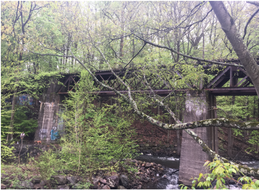
Photo 1: East Elevation, looking west.
